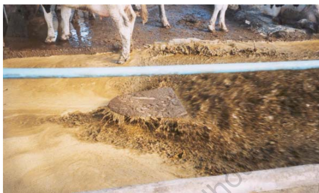
Flush wash valve centred on an internal passage, discharging recycled liquids.
