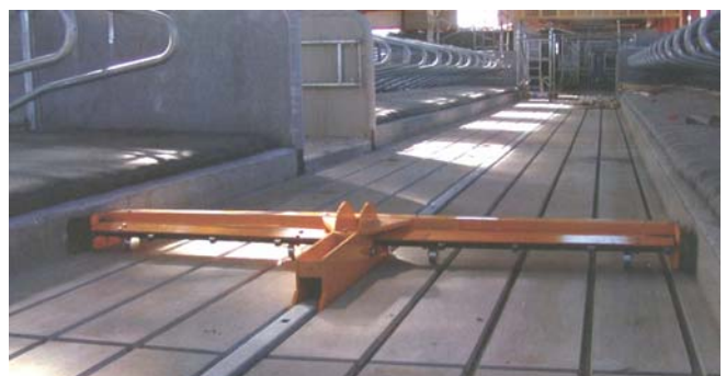
Completed slotted drained floor with scraper.
