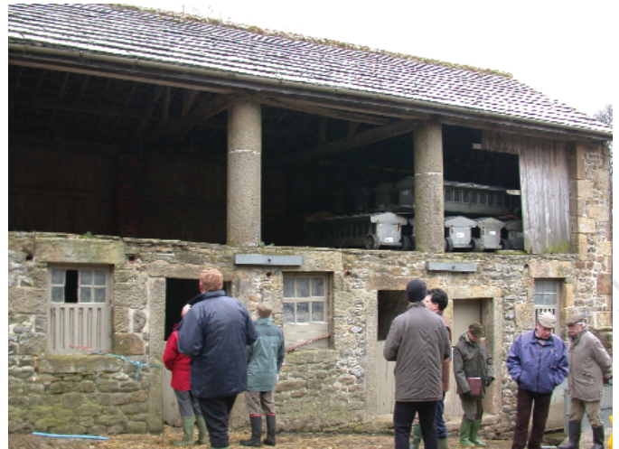
A lovely old barn which has reused some of the columns from Bolton Abbey
