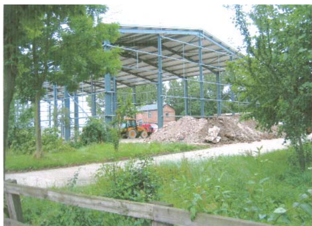
Potato store under construction
