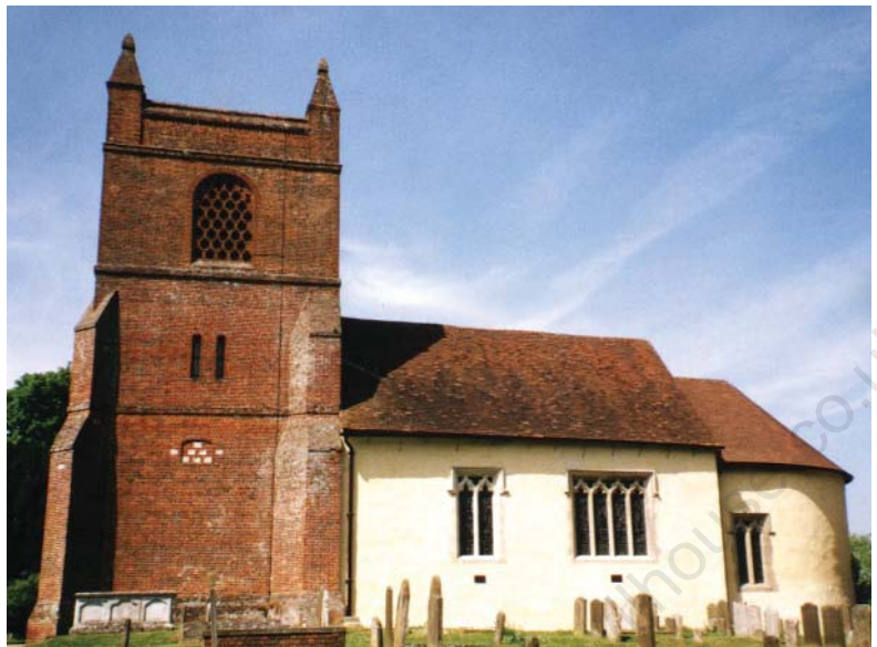
The church after completion of the work
