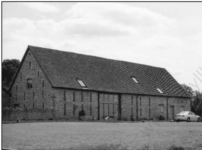
Barn conversion in Hereford which includes Central Extraction and Ventilation technology
