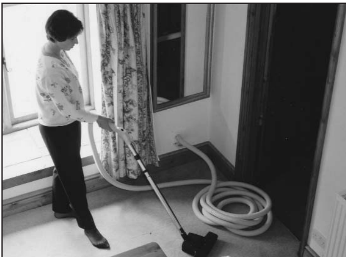
Showing the use of the Central Vacuum System in the Barn conversion in Hereford
