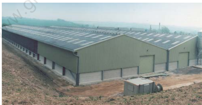
The 5000m 2 roof at the research facility in Berkshire - Designers - Scottish Agricultural Colleges' Design services.
