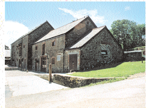
Barn Converted to restaurant.
